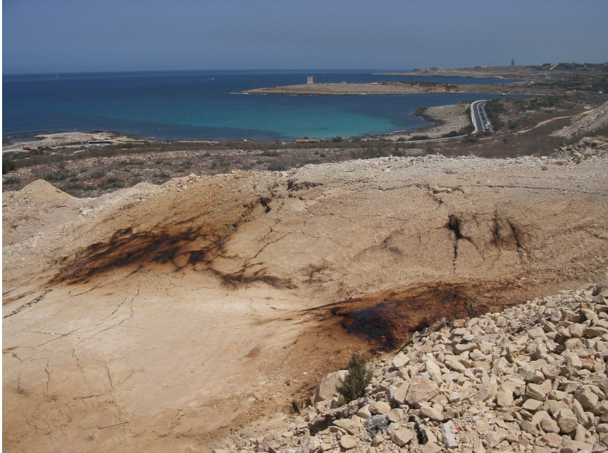
Plate 3.1: Combustion venting and waste settlement – Magħtab north face
